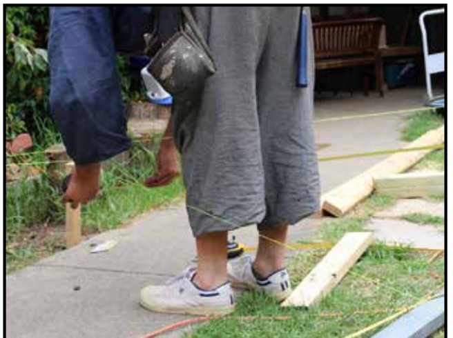
Liam and Osho Sama leveled the ground using traditional methods. Photograph: Katherine Yeo.
