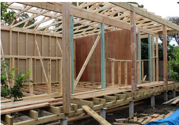
The framework sits in place. Photograph: Katherine Yeo
